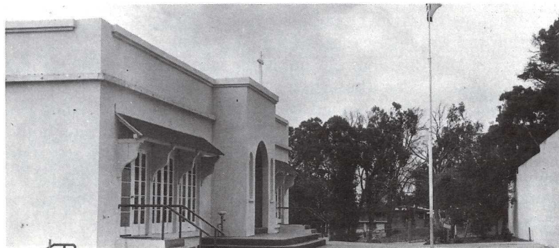
The old Del Mar Elementary School building became St. James Academy. Following the Academy's move to Solana Beach in 1972 it was purchased by the city and renovated and is presently Del Mar's City Hall.
